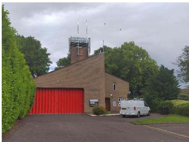
Charlbury Fire Station
